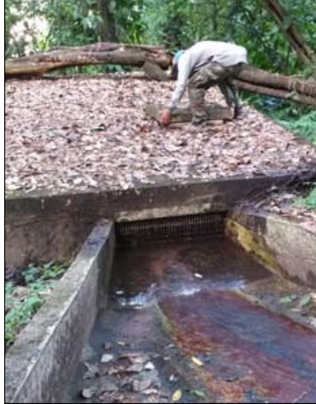
Las Flores receives its water from an intermittent spring-fed stream where water is captured (right) in a 27 year-old basin. One Day Challenge funds will be used to construct a storage tank and 700m of trenched pipe to bring a more reliable supply of water to the community.
